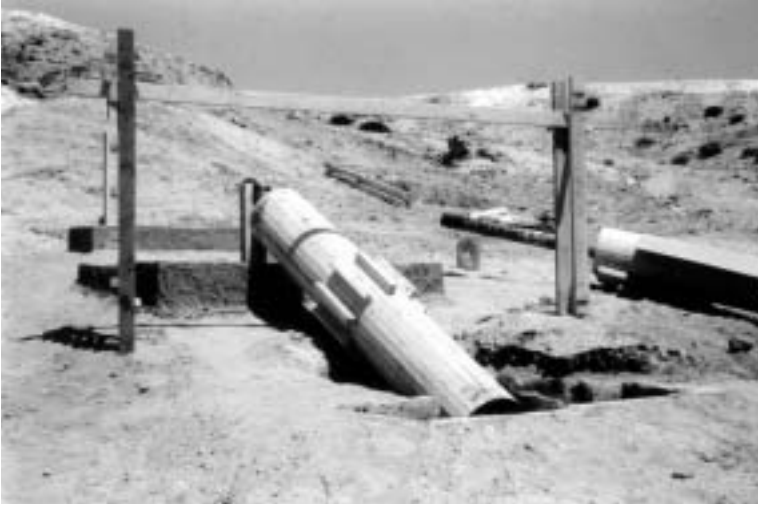
FIG. 5 The BBC water screw, complete and mounted. (Photo by John Peter Oleson.)
